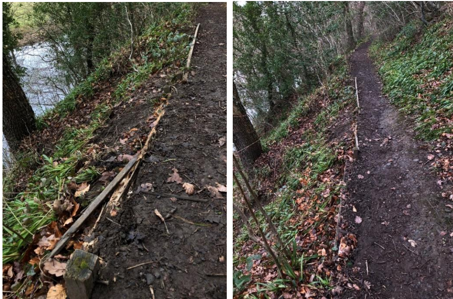
Path revetment before works
