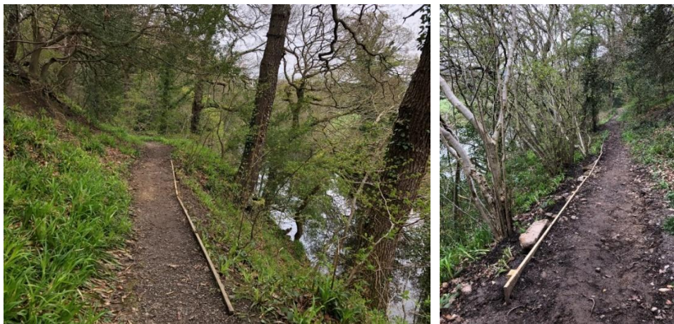
Path improvements after works
