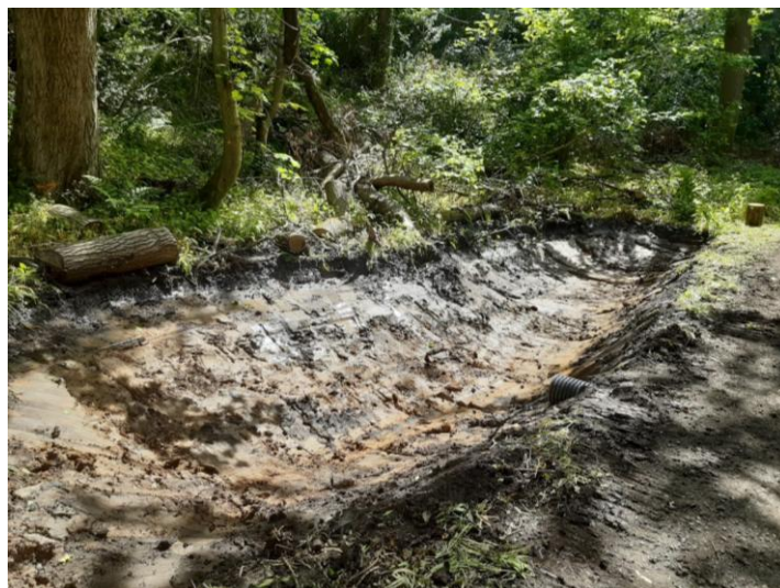
Pond excavation in summer 2022
