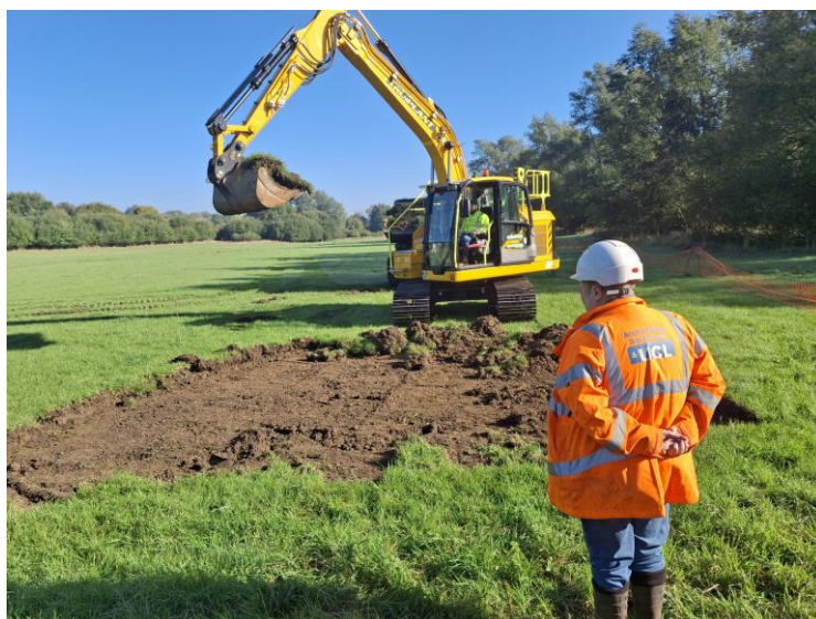
Digger breaking ground at Fiddler's Hill
