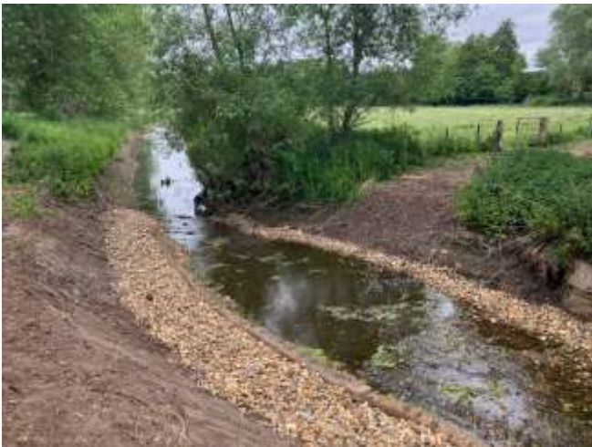
Photo of new channel and Weir removal at site 2 and 3
