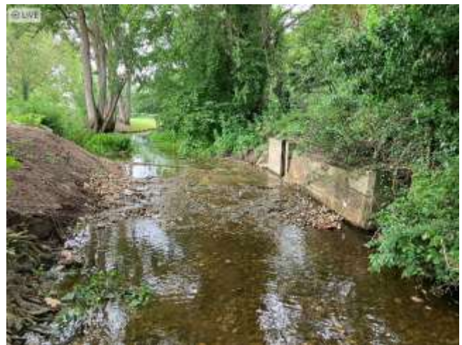
Photo of new channel and Weir removal at site 2 and 3
