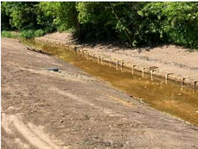
Creation of two stage channel
